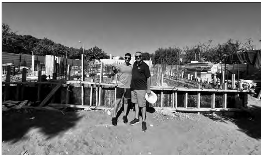
Left: Mike Averbach, left, and Michael Sachs at the construction site of the Vancouver/Winnipeg-supported women's shelter in Israel.
